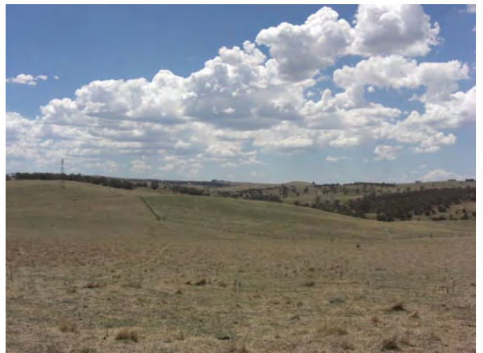
6. Transmission line from highest point
