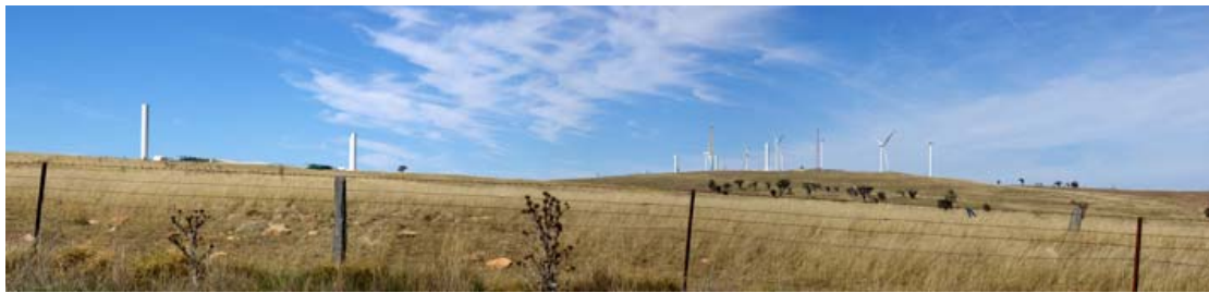
Plate 8. Illustrating general construction activities at the Capital Hill wind farm site, including views toward cranes, partial construction of towers and laydown areas.
