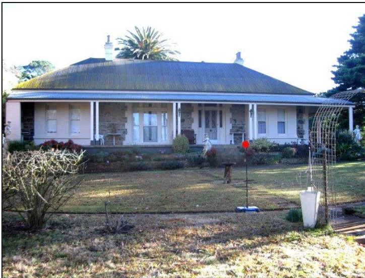
Figure 21 Leeston Measurement Location
