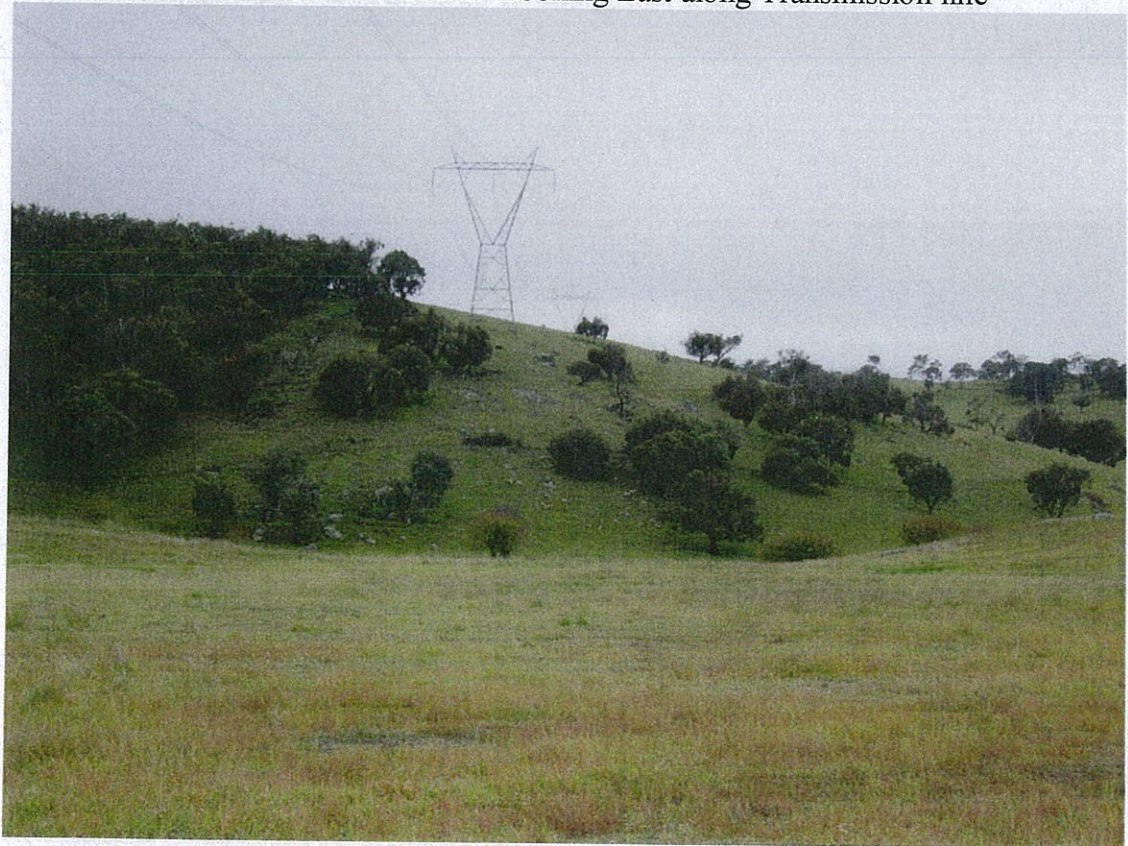
South Site: Photo Point J - Looking East along Transmission line
