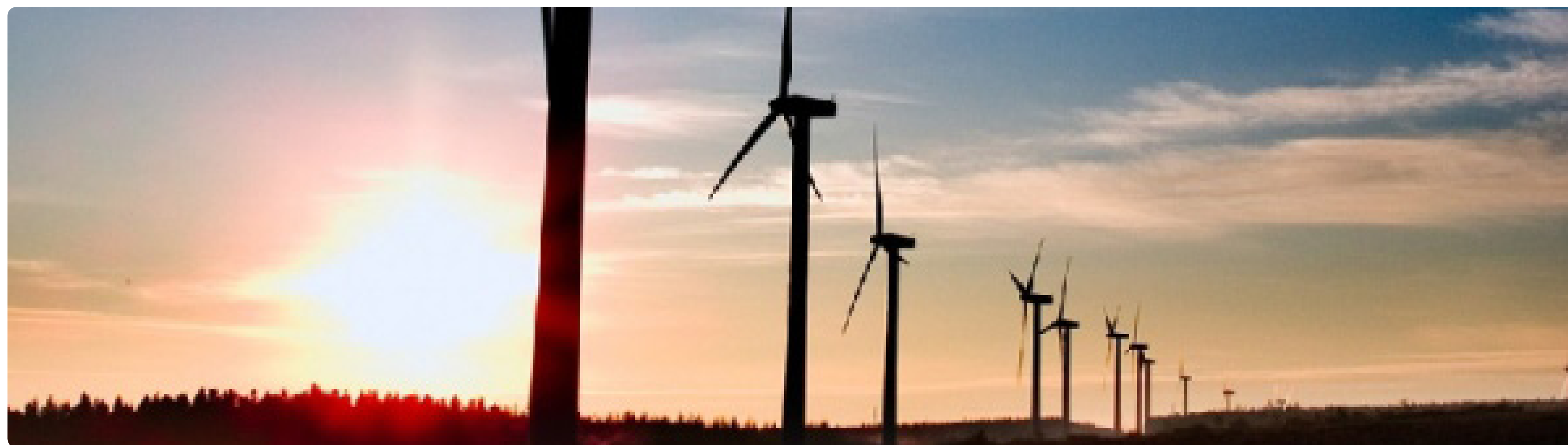
International example of a wind farm
