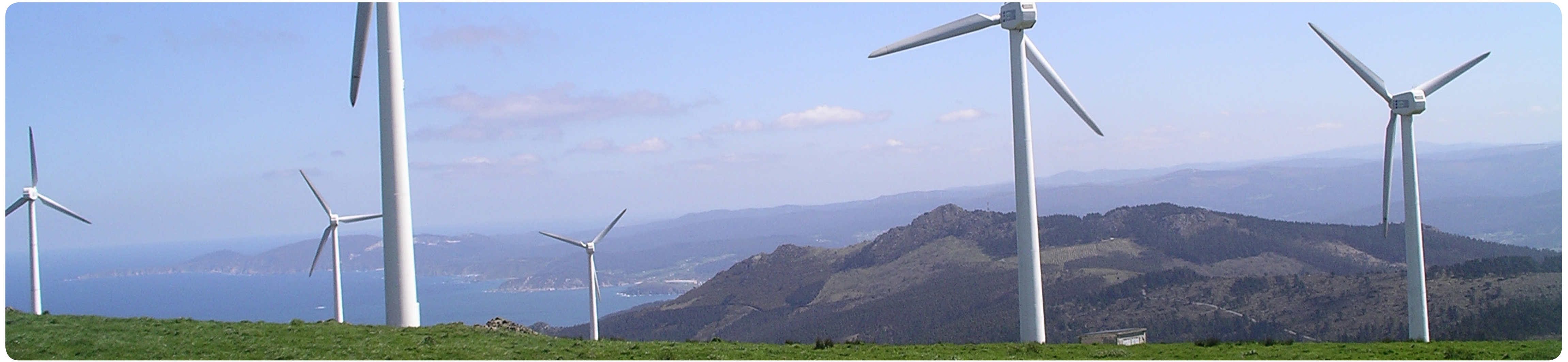
International example of a wind farm
