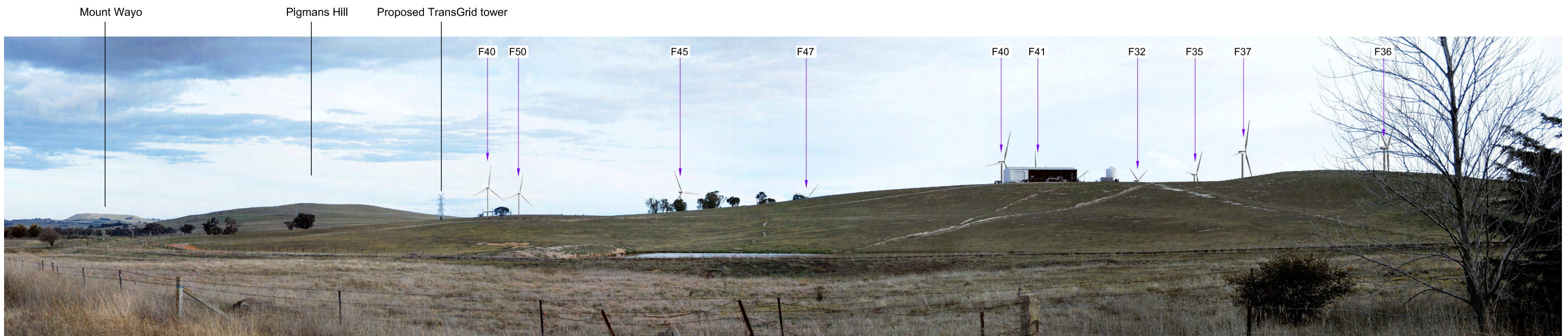
Photomontage 8b Woodhouselee Road - View south to west south west from Woodhouselee Road toward the C2WF Mod-2 layout. This photomontage illustrates the proposed C2WF Mod-2 wind turbine layout at the 160 metre tip height.
