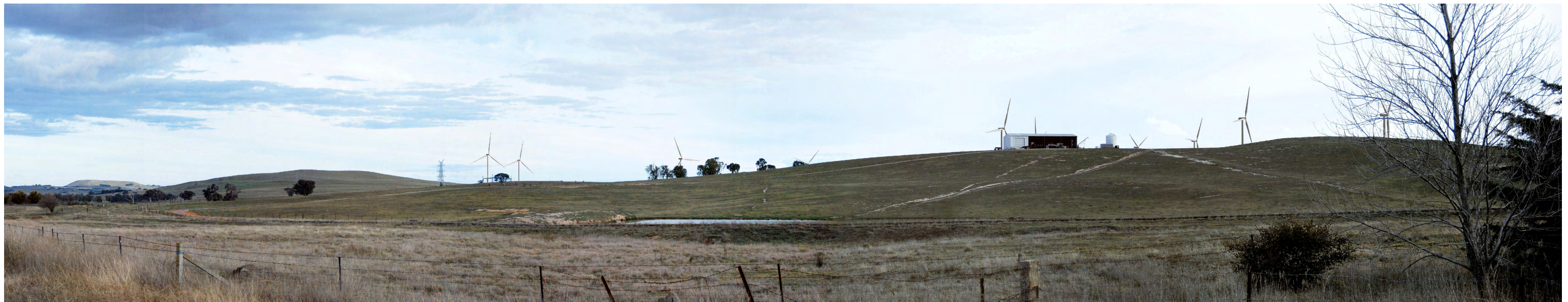
Photomontage 8d Woodhouselee Road - View south to west south west from Woodhouselee Road toward the C2WF Mod-2 wind turbine layout. This photomontage illustrates the proposed C2WF Mod-2 wind turbine layout at the 160 metre tip height.
