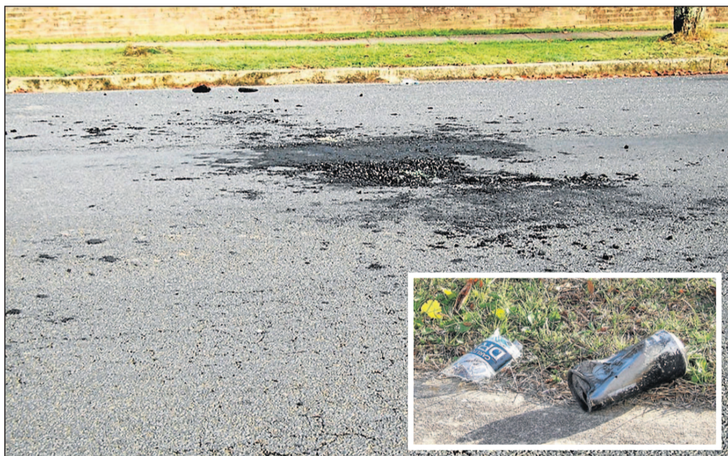
• What is left over of the fire lit on Kialla Rd during the early hours of Saturday morning. Inset: Broken glass was spread over a wide area on both sides of the street.
