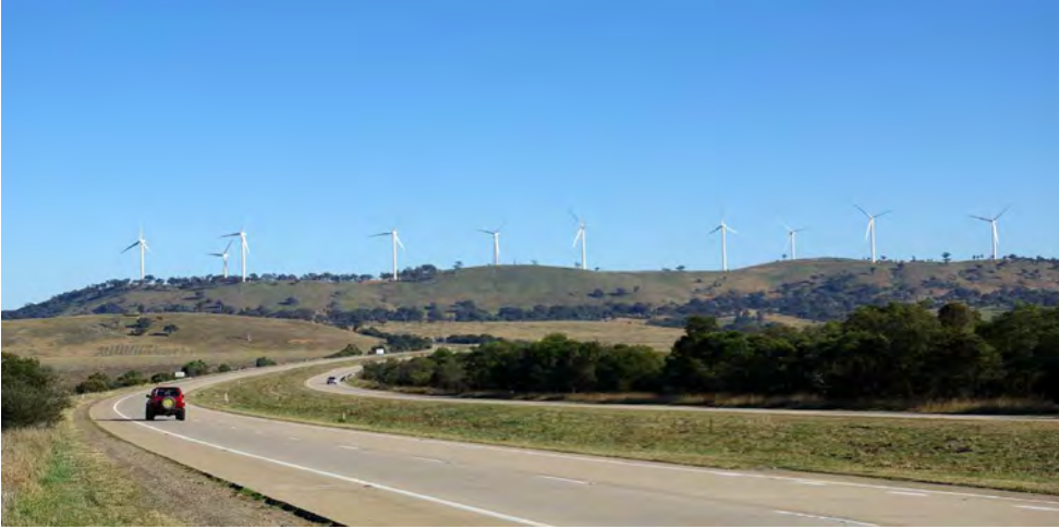
PHOTO A - DAY TIME VIEW FROM HUME HIGHWAY TOWARD CULLERIN WIND FARM AT AROUND 3.5KM (13th June 2010)
