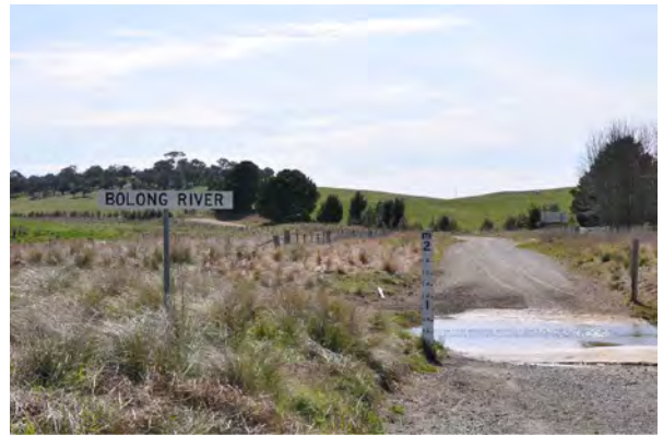
Photo Location TL10- View north along Tyrl Tyrl Rd
