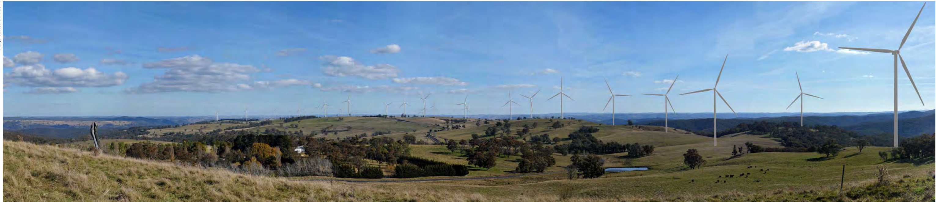
Photomontage Location PM 6 Hutton Hill Proposed view, extended panorama south south west to north west (Bearing 195° to 320°)
