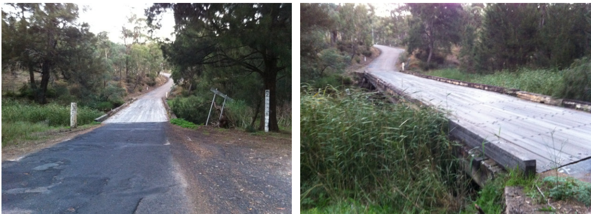
Plate 3-1 Abercrombie River Crossing (South of Paling Yards Site)
