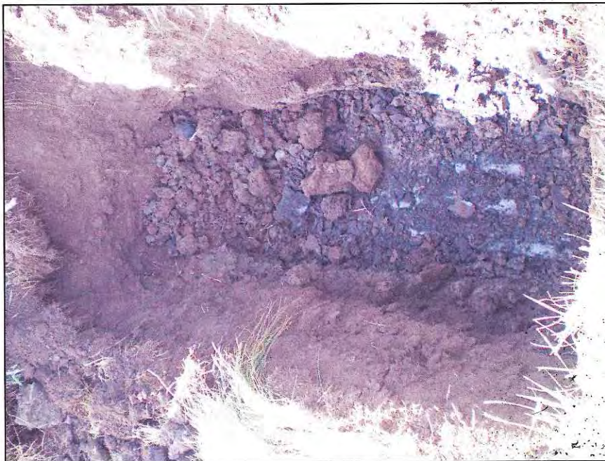
Test Pit TP56
