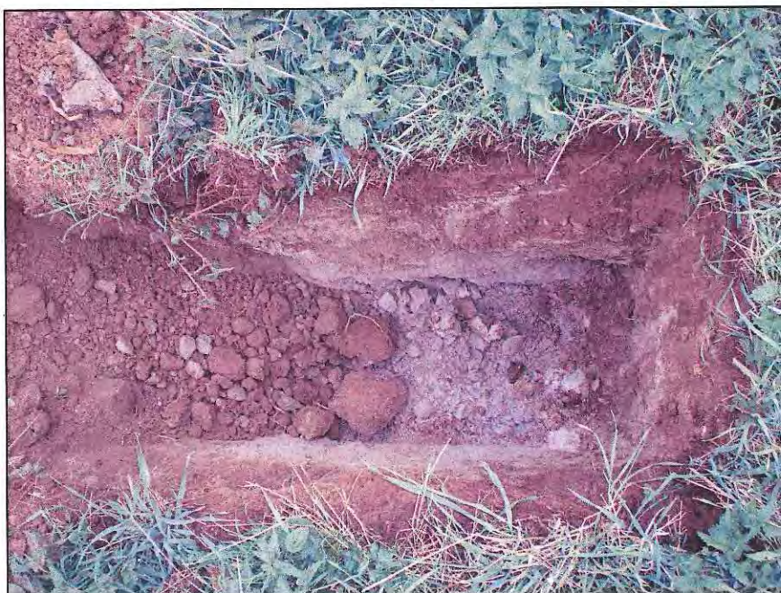
Test Pit TP23
