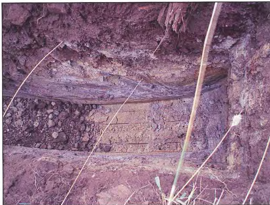
Test Pit TP08
