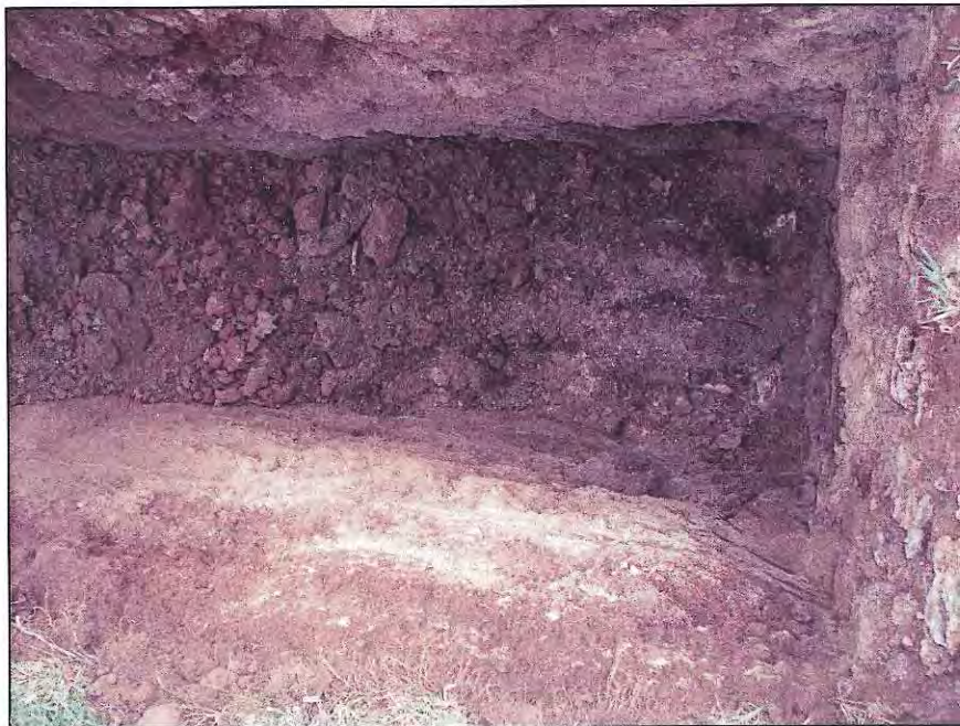
Test Pit TP33
