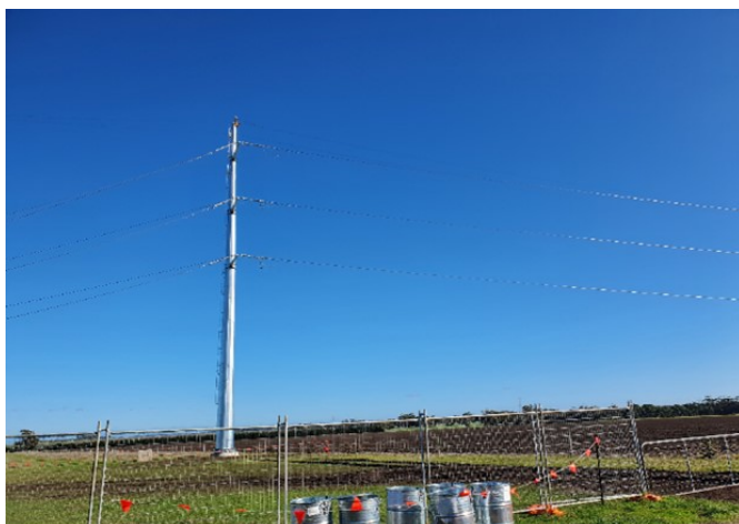
(Pictured) Preliminary stringing of Transmission Line
