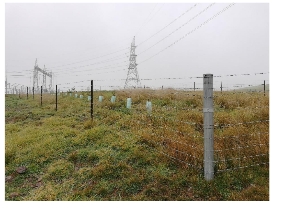
PA4 – Taken from NE corner (facing south)
