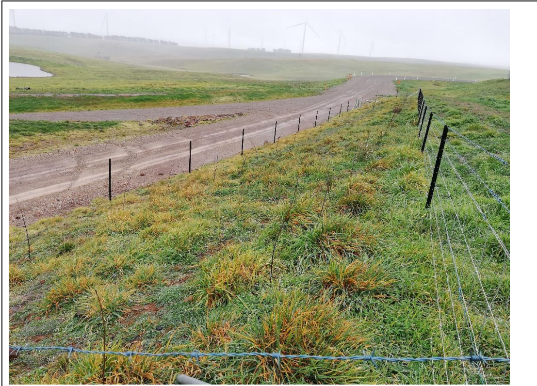
PA5 – Taken from SW corner (facing east)
