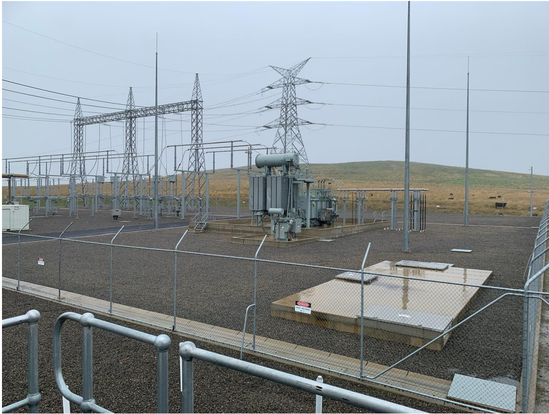
Substation transformer bund
