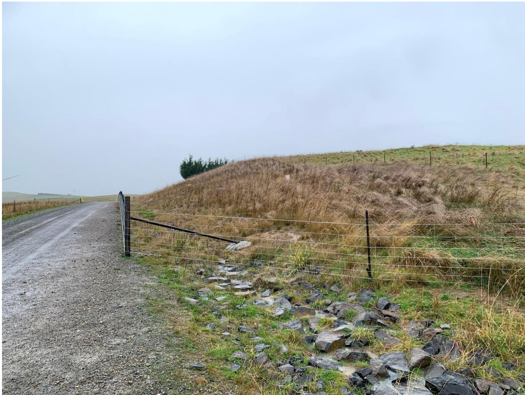
Fenced screening planting and permanent drainage works
