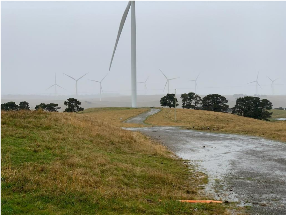
Internal Access Road
